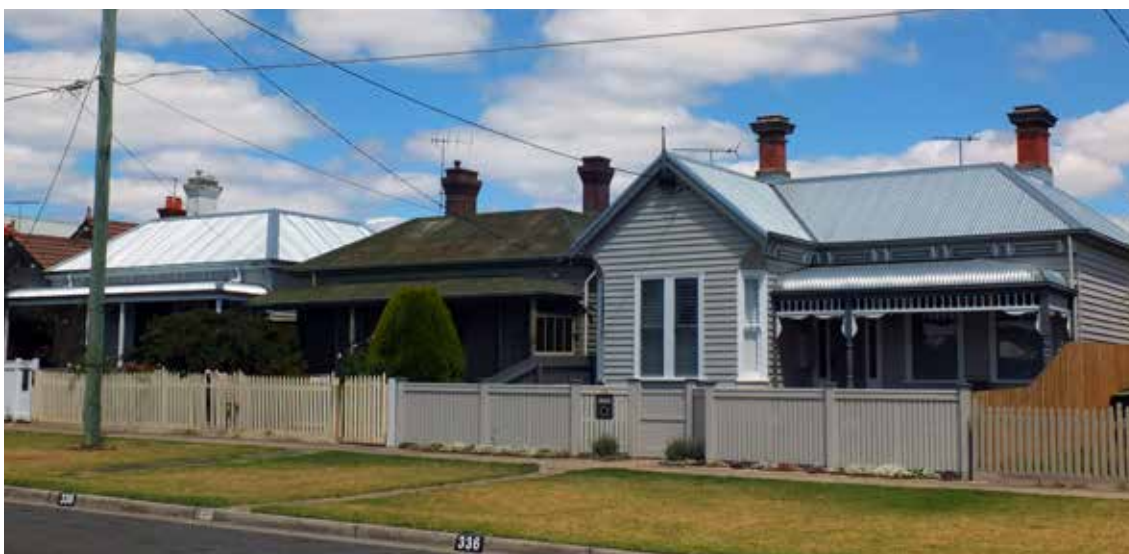
Figure 38 Streetscape, East Geelong. A Victorian dwelling (left) with a new Zinalume® roof and a Late Victorian dwelling (right) with a new galvanised steel roof.
