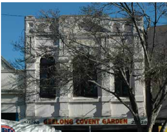
Figure 36 Geelong Covent Garden, Moorabool Street, Geelong, showing introduced overpainting to the facade and the introduced shopfronts and verandah.
