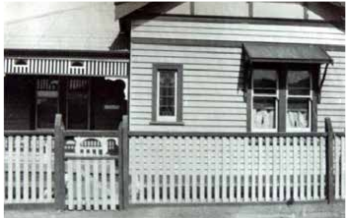
Figure 77 Edwardian styled dwelling having a timber picket fence with a simple capping.
