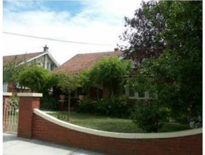
Figure 85 Interwar solid brick fence, being sufficiently low not to obstruct the view to the front garden.
