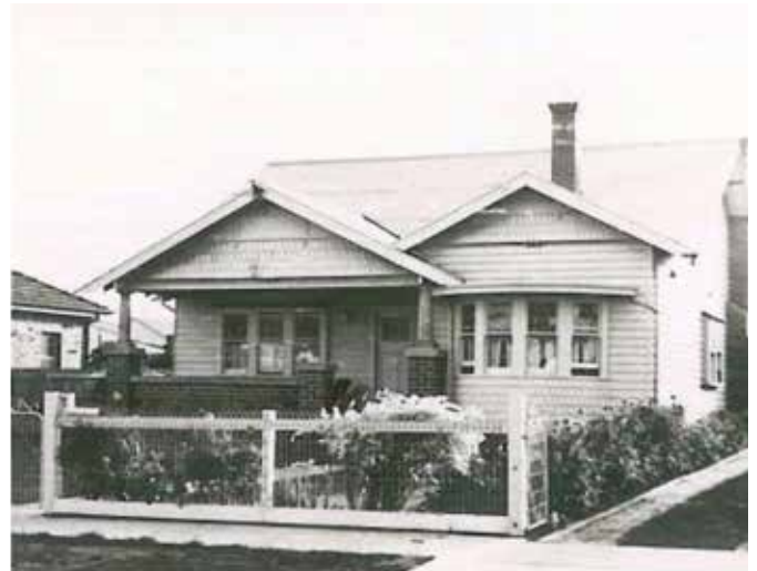
Figure 83 Timber post and rail, and woven wire fence to an interwar bungalow styled dwelling.
