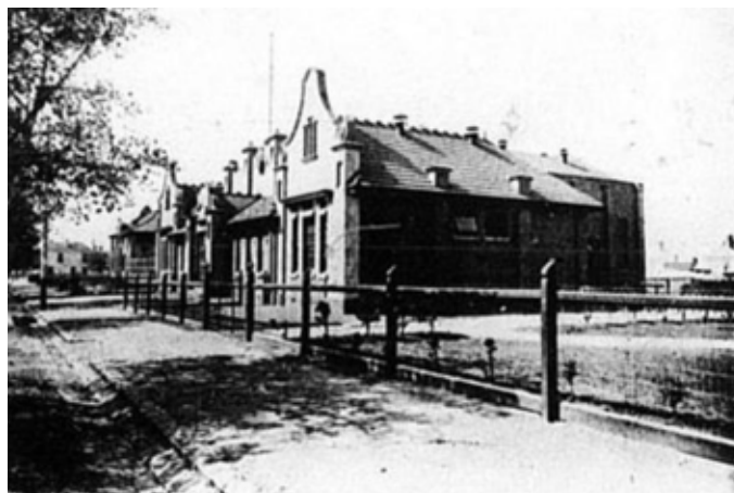
Figure 79 Capped timber post and woven wire fence. Source: News of the Week, 1916.
