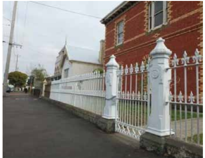
Figure 72 Substantial late Victorian brick dwelling with iron palisade fence having cast iron piers and bluestone plinths.
