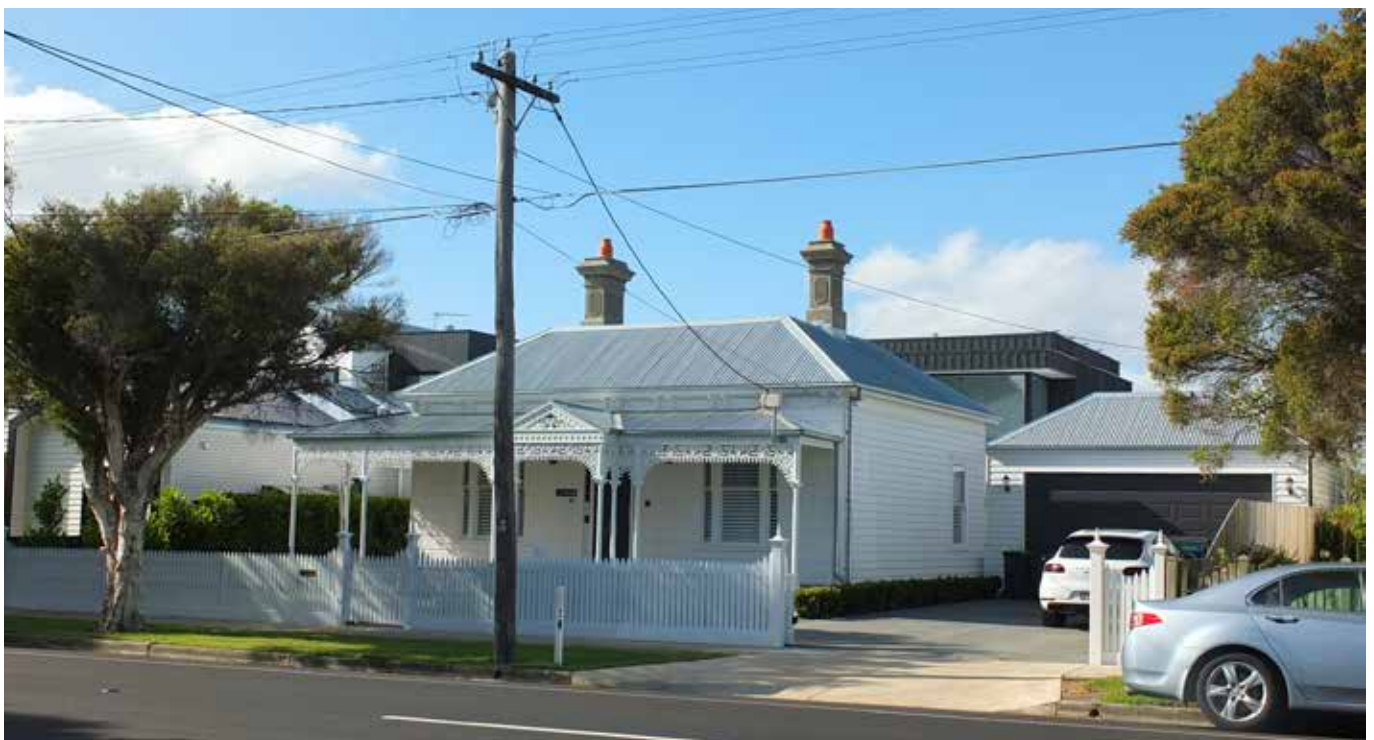
Figure 16 Dwelling, Geelong West. Contemporary two storey additions as a separate entity at the rear with minimal visibility from the street. The garage is recessive and is a contemporary interpretation of the dwelling given its exposure at the front.
