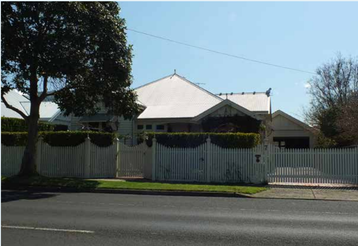
Figure 40 Dwelling, Drumcondra. A recessive garage to a dwelling.
