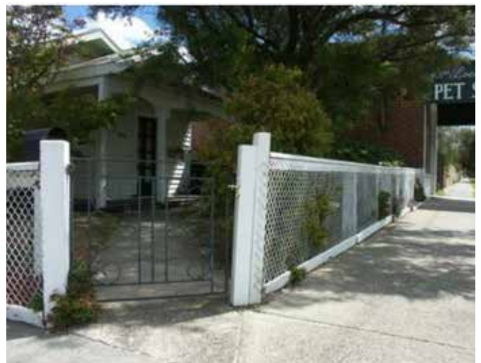
Figure 84 Interwar bungalow styled dwelling with a capped timber post and chain mesh front fence having open geometric steel gate.
