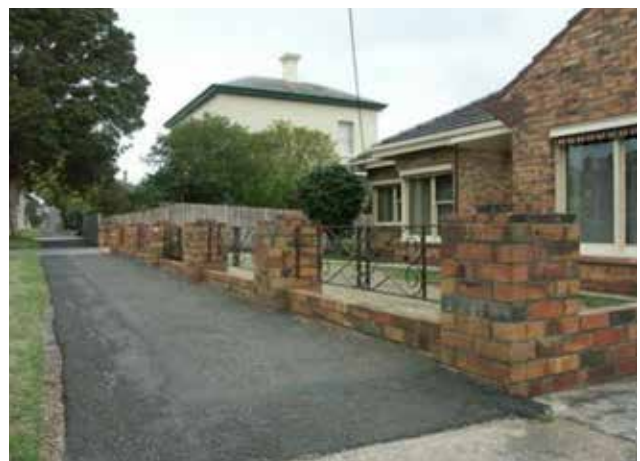
Figure 87 Low solid brick fence with open bays with trussed geometric panels.
