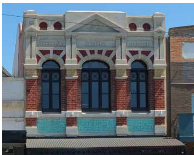
Figure 37 Geelong Covent Garden, Moorabool Street, Geelong, showing the exterior as largely originally intended. The overpainting was removed by approved poultice method, leaving the surface of the brickwork and tiles undamaged.
