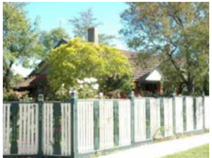
Figure 82 Capped timber picket fence to an interwar bungalow styled dwelling.
