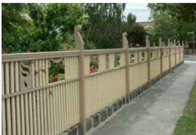
Figure 76 Details of Federation era picket fence with fretwork capping.
