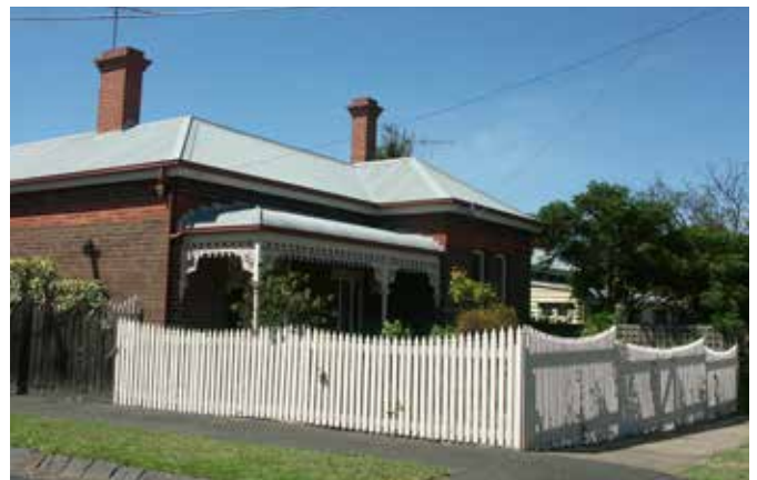
Figure 70 Late Victorian styled brick dwelling with pointed timber picket fence.
