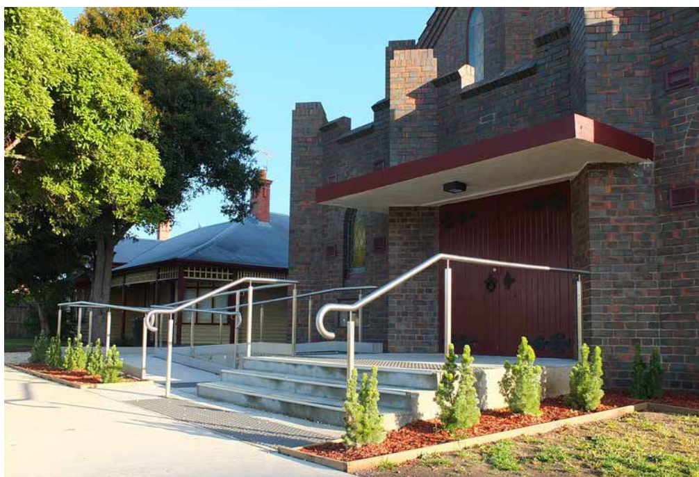
Figure 48 Former Shenton Methodist Church (now part of Geelong High School), Geelong. New ramp and stairs added for accessibility.
