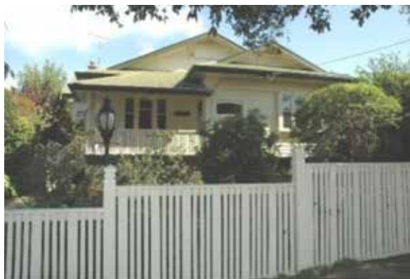
Figure 90 Fence stepped along slope of boundary.
