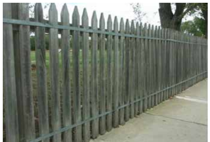
Figure 71 Unpainted timber picket fence with hoop iron used to reinforce the pickets
