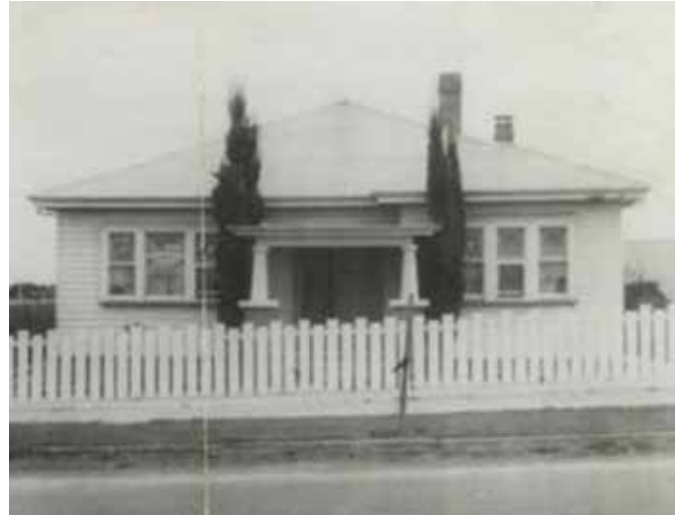
Figure 81 Flat timber picket fence to an interwar bungalow styled dwelling.
