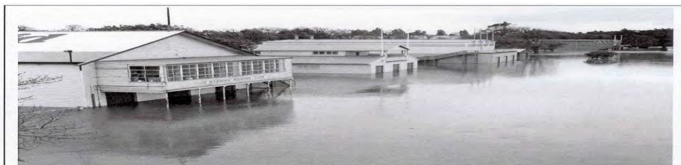
Rowing clubrooms, Barwon Tce, 1983
