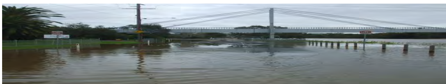
Barrabool Road & McIntyre Footbridge 2011
