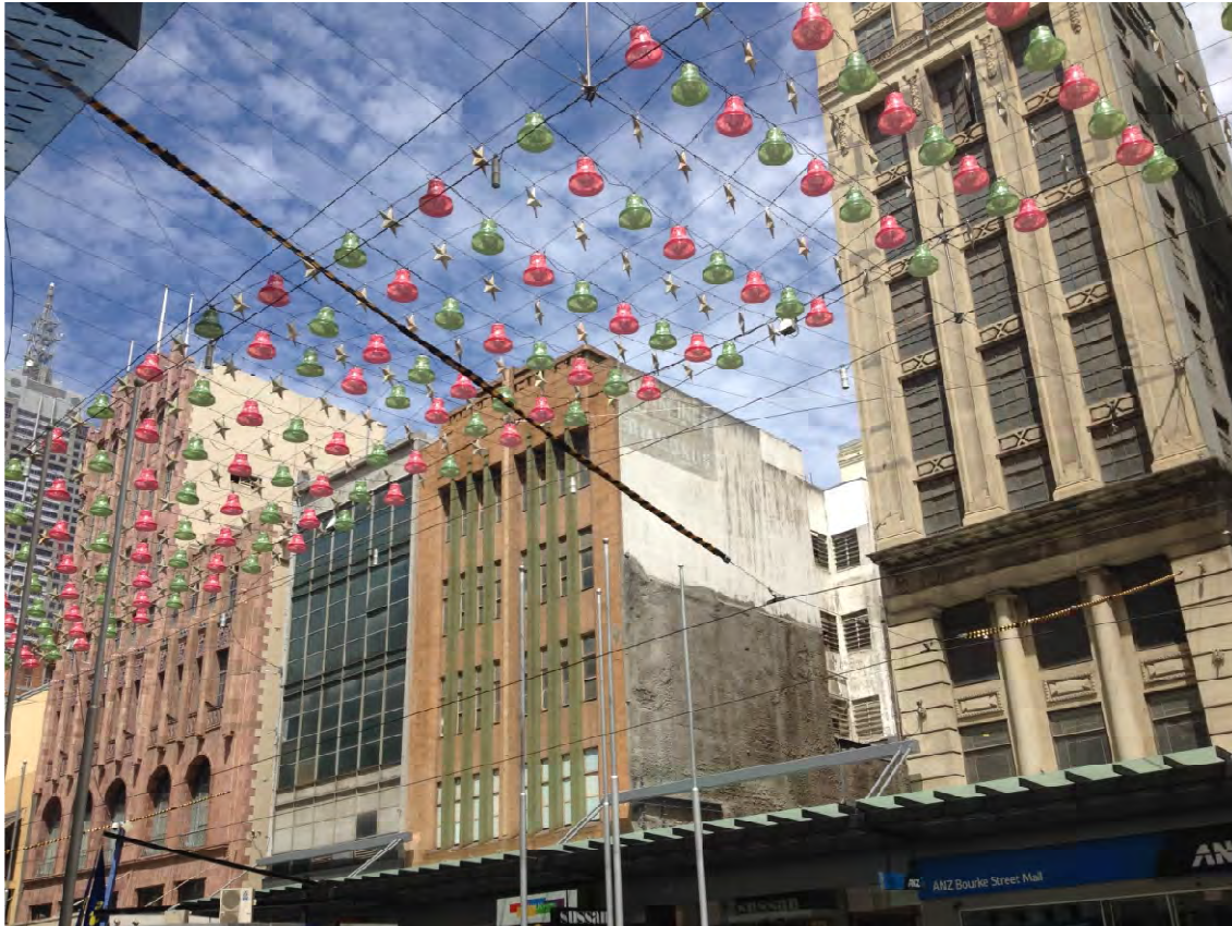
Bourke Street Mall Catenary Lighting Example
