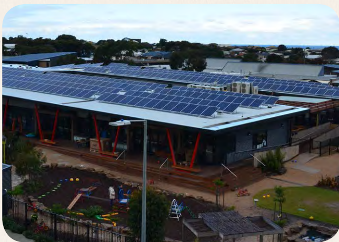
Boorai Centre Ocean Grove: 80kW solar system
