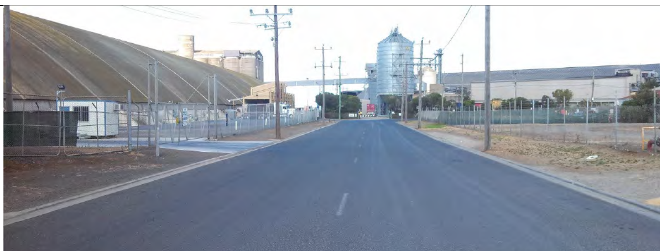
McLeod Street (Looking East – site on right) Source: ESR Transport Planning
